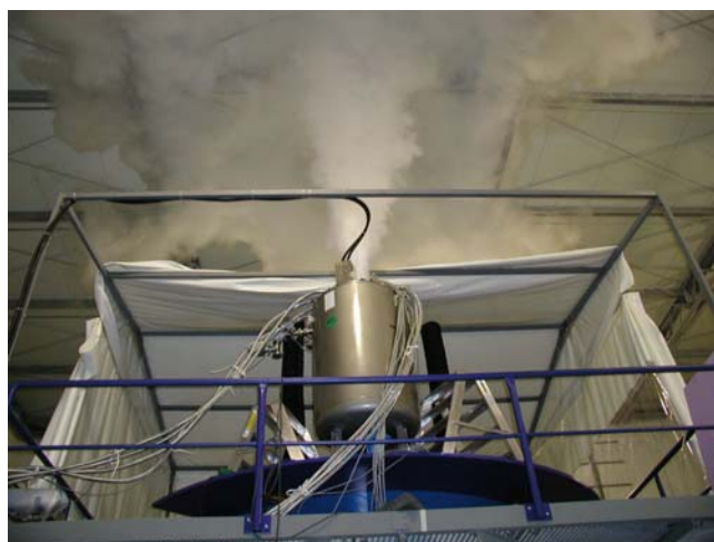
Fig. 7: Supply cryostat with the exhausting helium gas at the quench.
