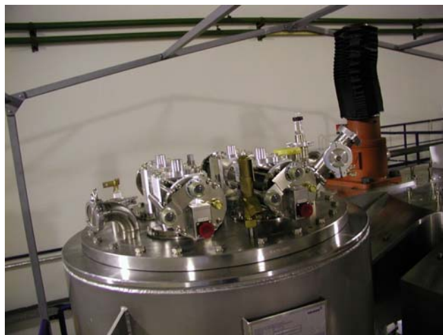
Fig. 5: The supply cryostat with four cold heads and instrumentation.
