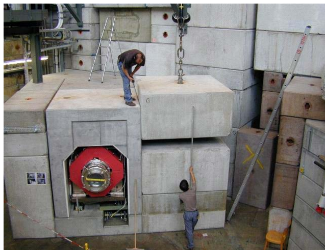
Fig. 5: The beam line components following the insertion wagon are also packed in concrete blocks. The blocks in the background are part of the primary shielding.
