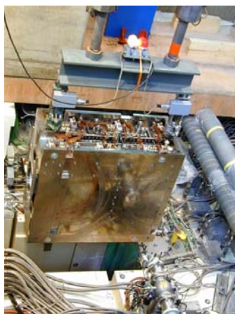
Fig. 4: The solenoid was installed at the end of April 2004. It was attached to the revolvable crane hook using special remote-controlled equipment. The radiation level around the production target prohibited direct access.
