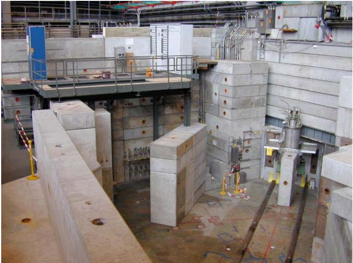
Fig. 5: The former \mu E4 area has been rearranged for the new beam line. In the background are the new platforms for the electrical cabinets. At the end of the rails the insertion wagon with the cryostat of the muon channel can be seen.
