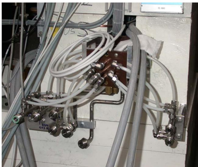
**Fig. 10:** The power and cooling water connections for the first QSM triplet and the ASR61 bending magnet.
